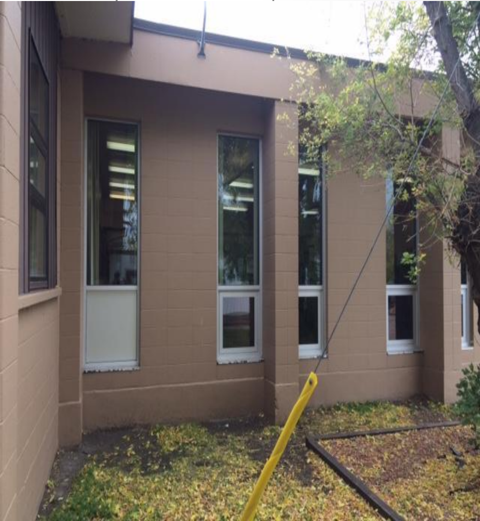
Library Window Replacement
